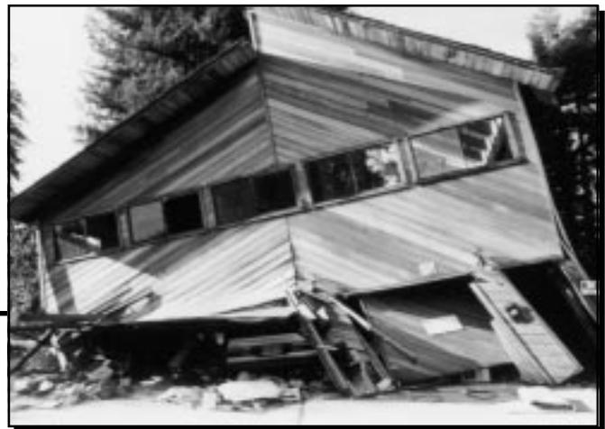
**This mountain home was built over a garage, and its walls were not strong enough to withstand an earthquake.**
