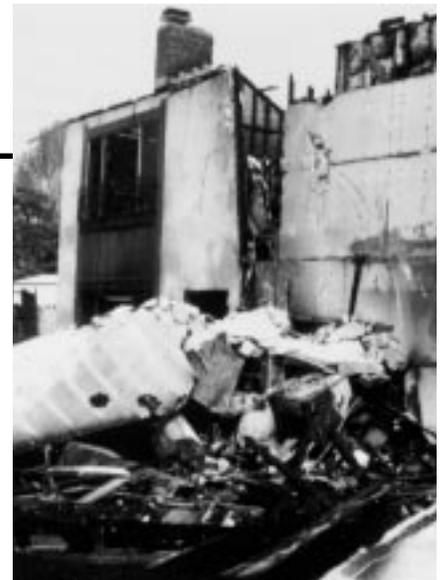
**The unbraced water heater in this home fell during an earthquake; the resulting fire destroyed the home.**
